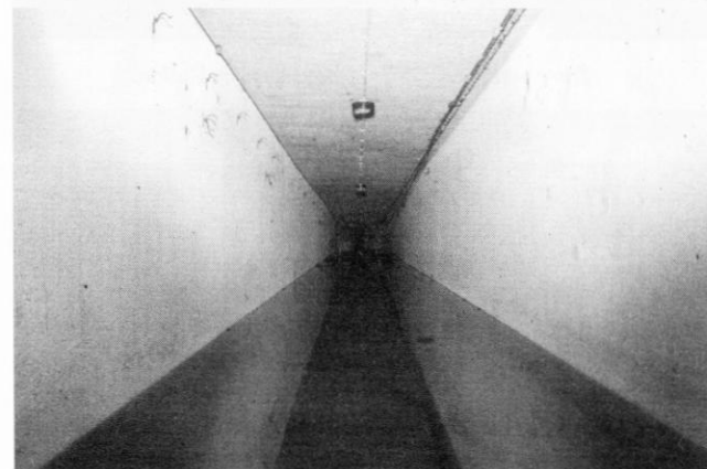
The entrance tunnel halfway through pumping. Photo by Gavin Saxby
